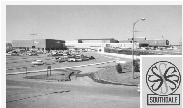
The 95-acre two-level Southdale Center Mall, with parking for 5,200 cars, opened on Oct. 8, 1956 in Edina, Minnesota, near Minneapolis. It was the country's first fully enclosed shopping center, with a constant temperature of 72 degrees.
